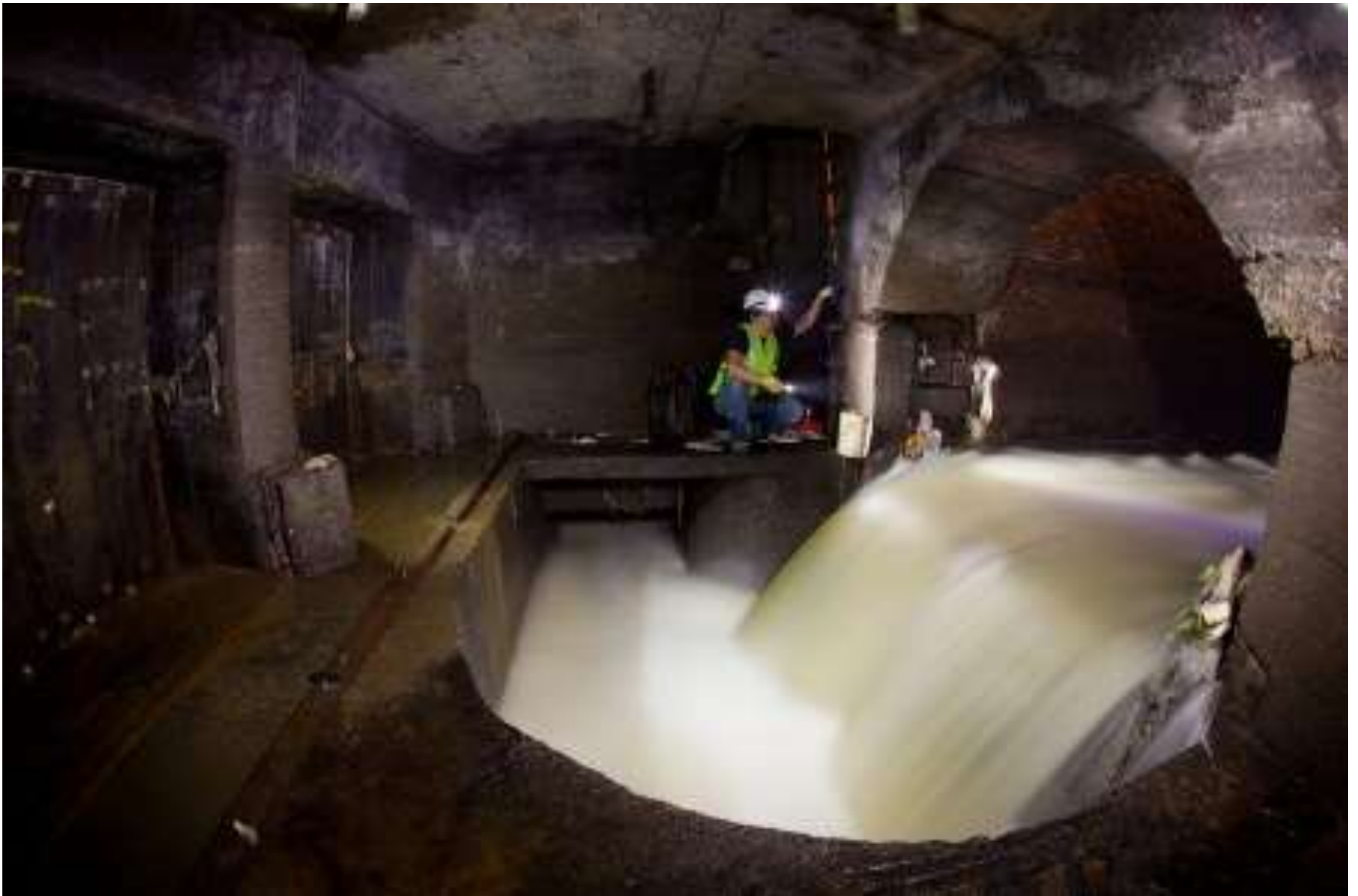
New York City “Combined Sewer Interceptor”
