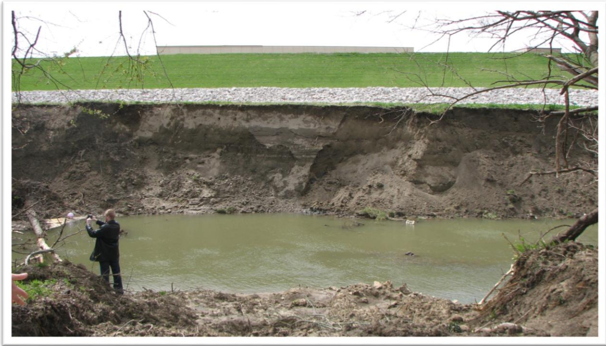
Figure 3-5: Bed degradation from the Missouri River moved up Line Creek in Riverside, Missouri causing damage to a major-federal levee. Note the rock toe of the levee at the top of the eroded bank.
