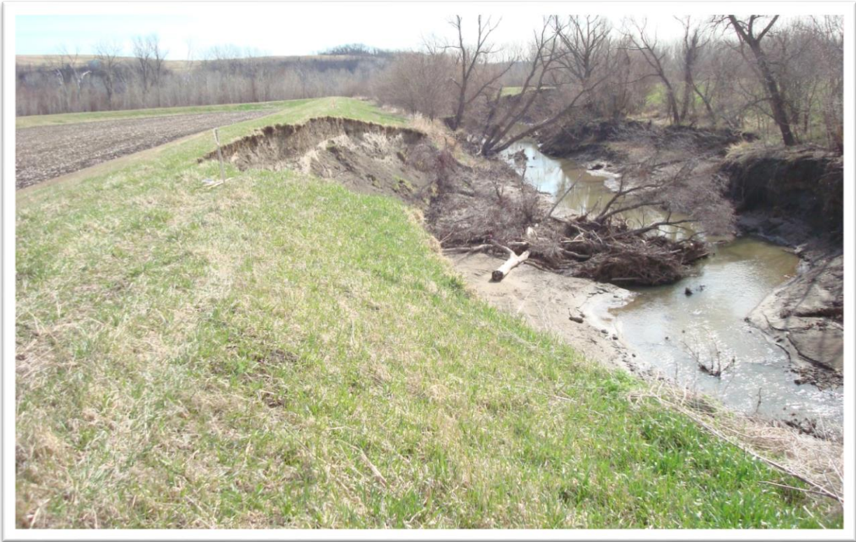
Figure 3-4: Bed degradation from the Missouri River moved up a small tributary in Wyandotte County, Kansas contributing to damage on a non-federal levee in 2009.
