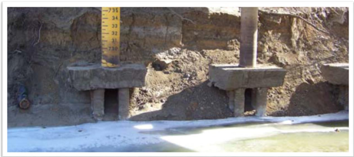
Figure 3-7: Bridge piers were damaged along a tributary to the Missouri River that was subject to bed degradation in Platte County, Missouri.
